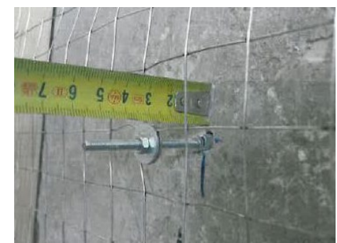
Electrowelded mesh fixing detail
