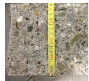
Concrete with Aeternum
